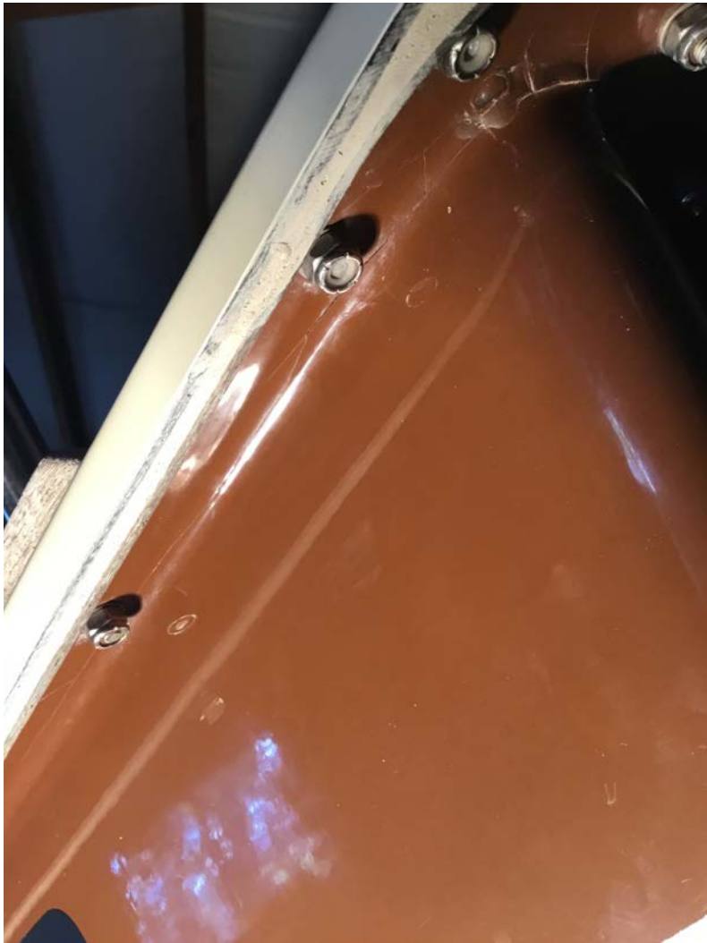
Starboard side crack extends ~9" aft (beyond last bolt)
